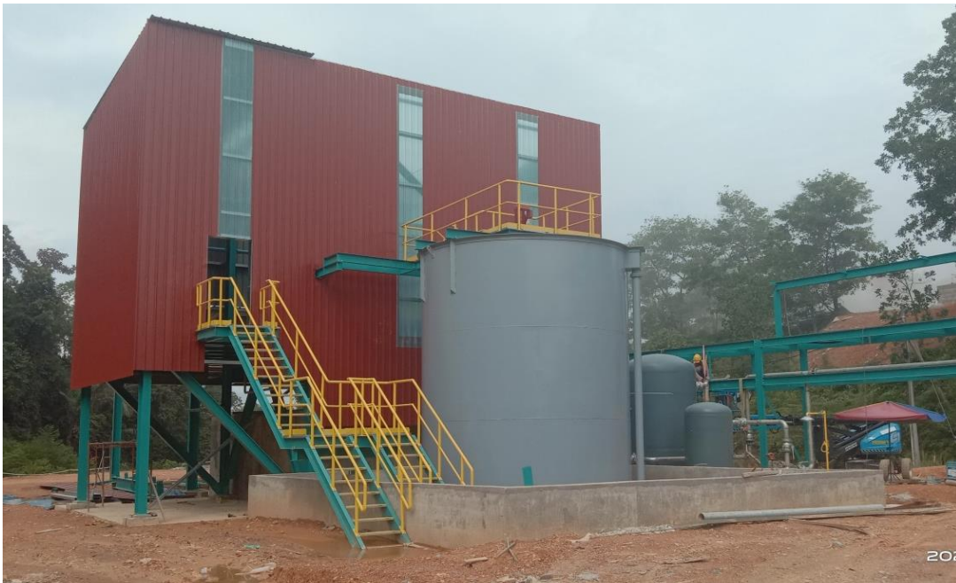
Figure 2: Concentrate Filter Building
