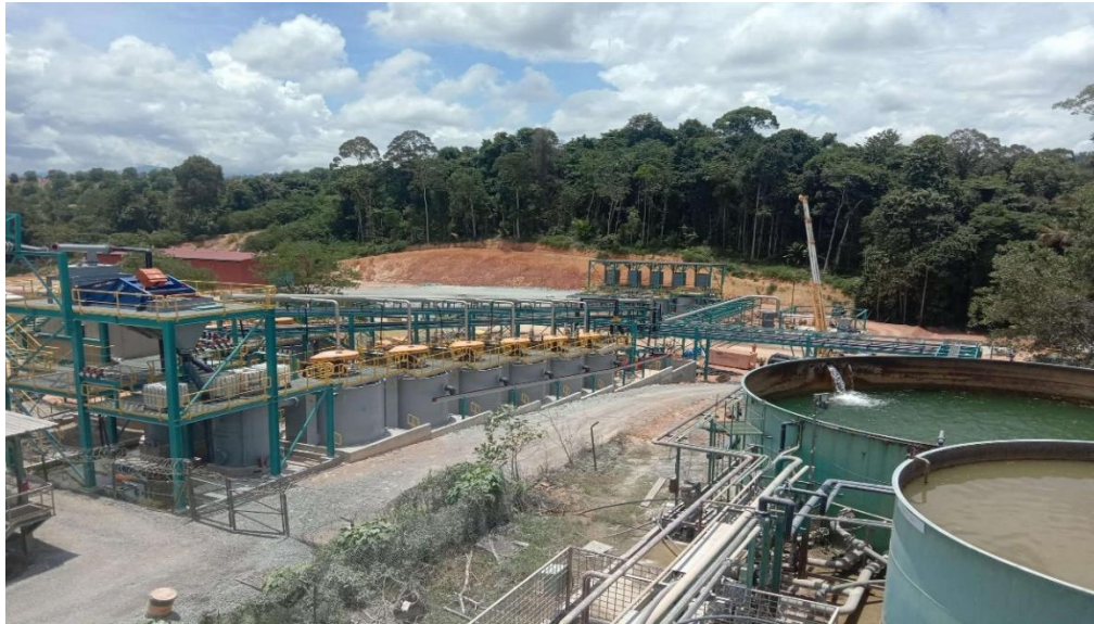
Figure 1: View of Flotation Plant Circuit Construction
