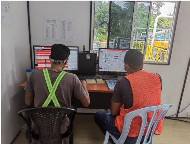
Figure 3: Operating Scada System
