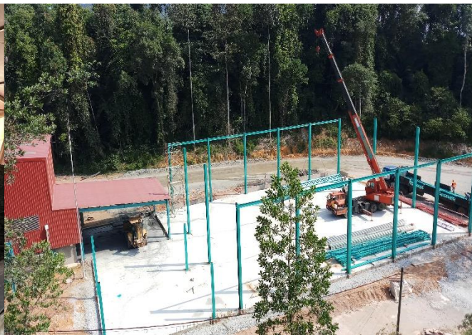
Figure 2. Concentrate Storage Construction
