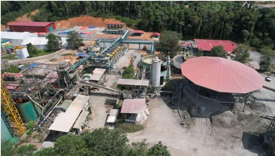
Figure 3: Selinsing Flotation Plant
