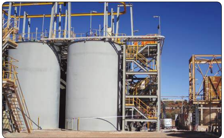
The processing facilities at the Murchison project in Western Australia.
