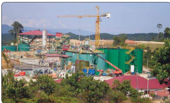
The Selinsing plant nearing completion of the expansion to an annual rate of 1 million tonnes.
