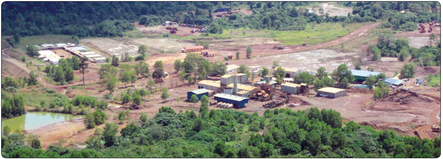
An overview of the facilities at the Mengapur Polymetallic Project.
